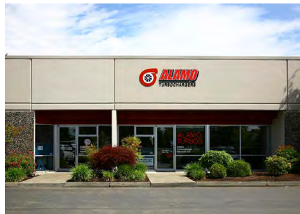
22737 - 72nd Avenue S. - Bldg C, #109 | Kent, WA
